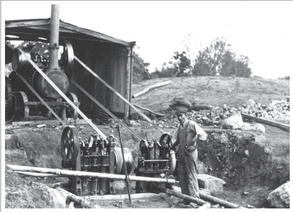
FIGURE 3.5: A portable steam-powered pumping system was used to pump water from the river.
