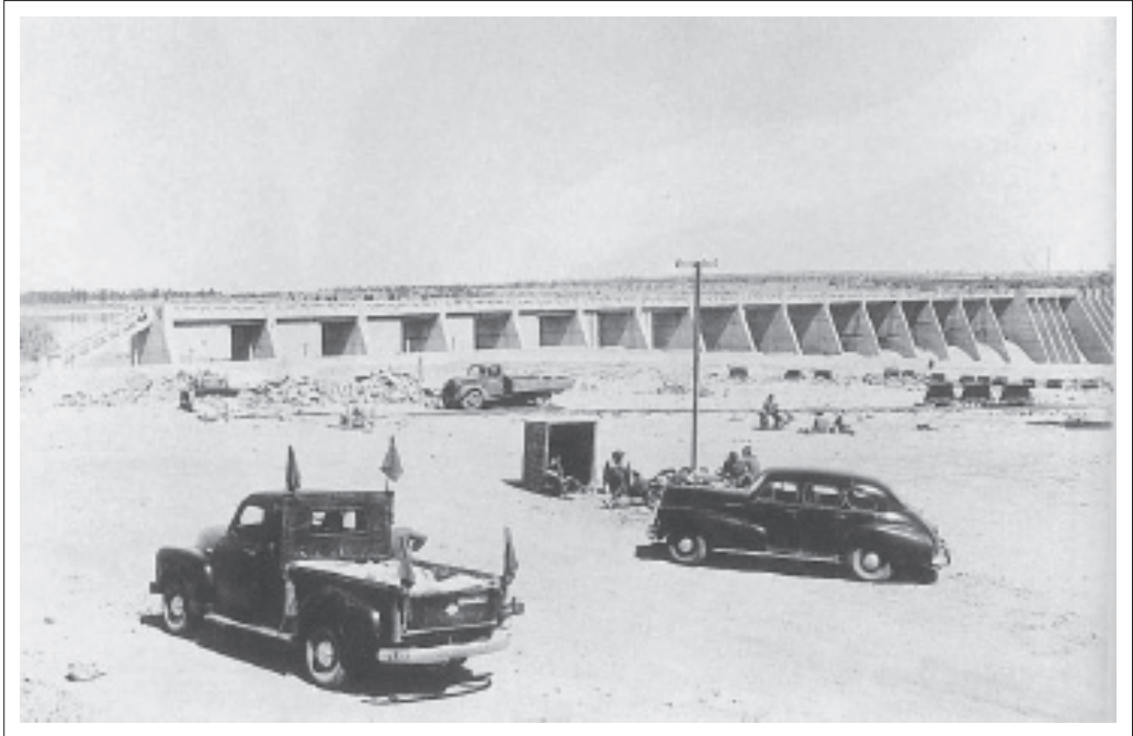
FIGURE 4.1: In 1950 the wall of the Vaal Dam was raised to secure a greater water capacity.
