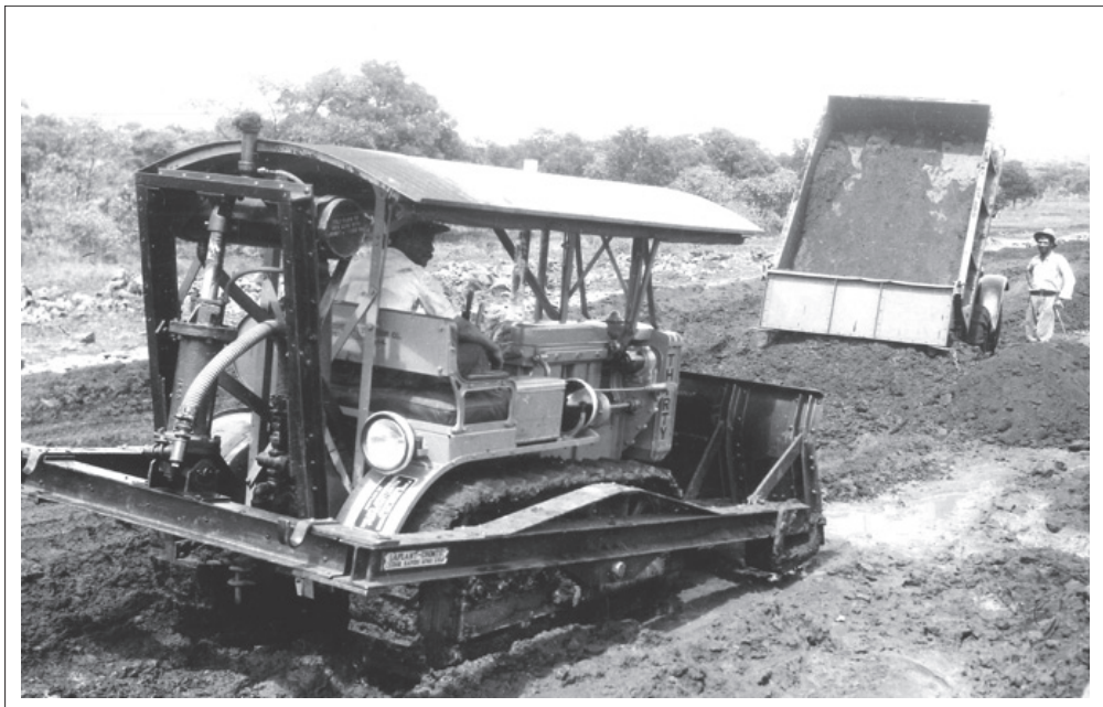
FIGURE 3.8: A Caterpillar 'Thirty' tractor bulldozer was used to level soil. In the background one of several tipping trucks used on the Marico-Bosveld Dam construction site.
